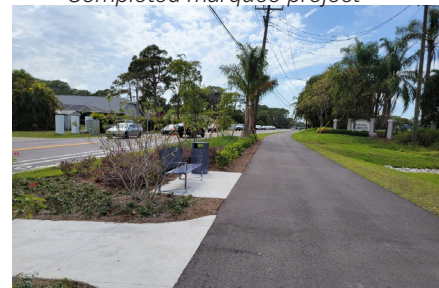
Completed marquee project
